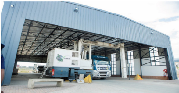
Non-Intrusive Equipment (Scanner) at Beitbridge Border Post
