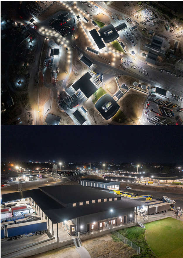
Aerial overview of the Beitbridge Border Post and the Freight Warehouse
