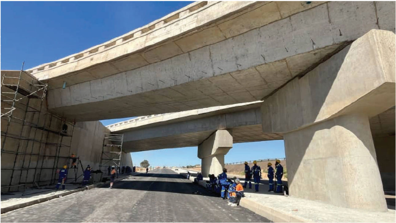
The Trabablas Interchange under construction, demonstrating the Government's commitment to using public revenue to develop infrastructure and build Zimbabwe.
